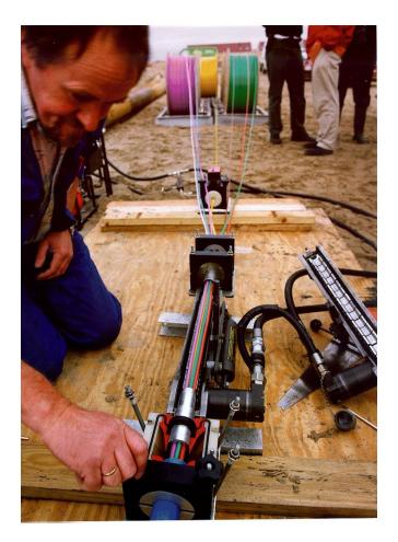
Figure 2 Installation of a bundle of guide-tubes in a protective HDPE duct by blowing
